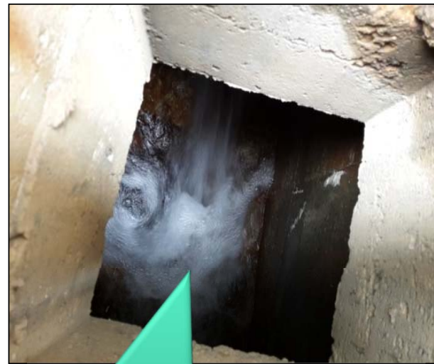
Visual Inspection: Water inflow to drainage manhole
