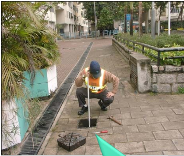
Sounding Inspection on valve by listening stick
